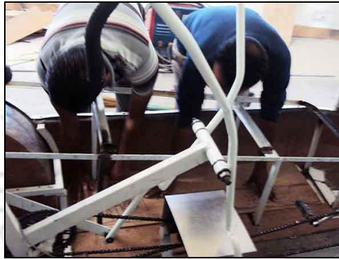
(c): Fixing the gaps between void areas of the catamaran hull.
