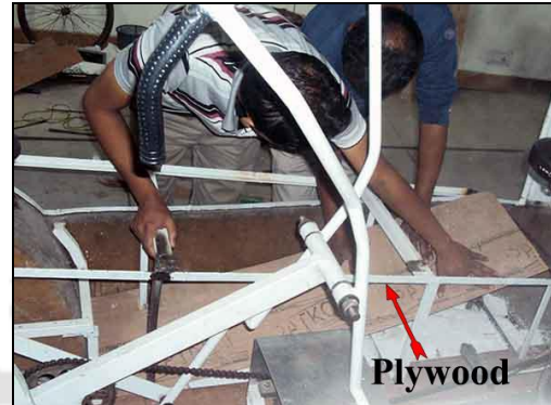
(b): 4 mm thick plywood placed on the void area after putting pour-in-place foam.
