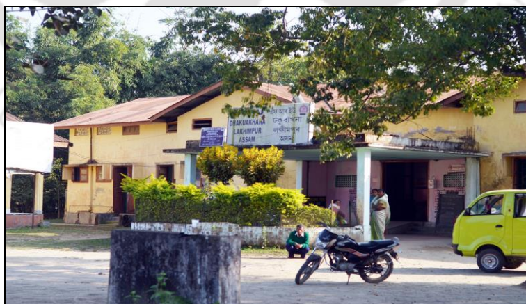
Figure 1.4: 30 bedded PHC in semi- urban areas. Source of Photograph: Author
