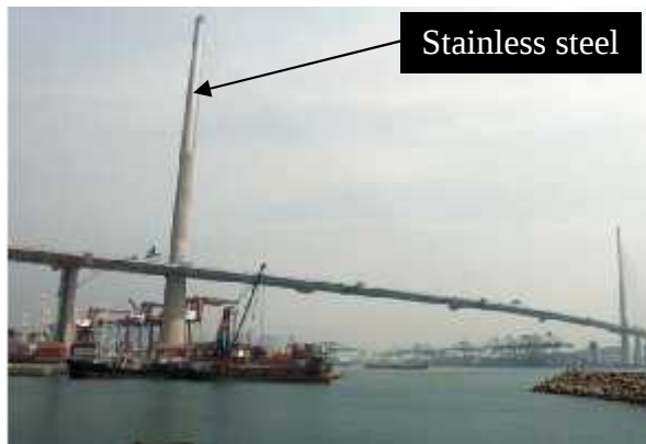
Figure 1.1: General view of Stonecutters Bridge ( www.worldstainless.org )
