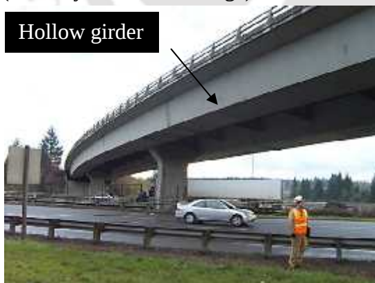
Figure 1.14: Kamal's Bridge in Tualatin, (www.campbellsci.com)
