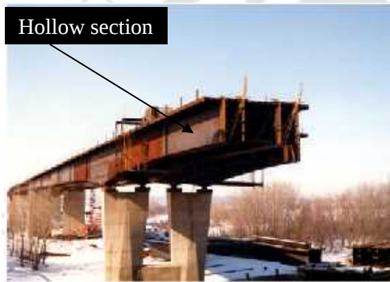
Figure 1.12: Illinois River bridge (courtesy. American bridge)
