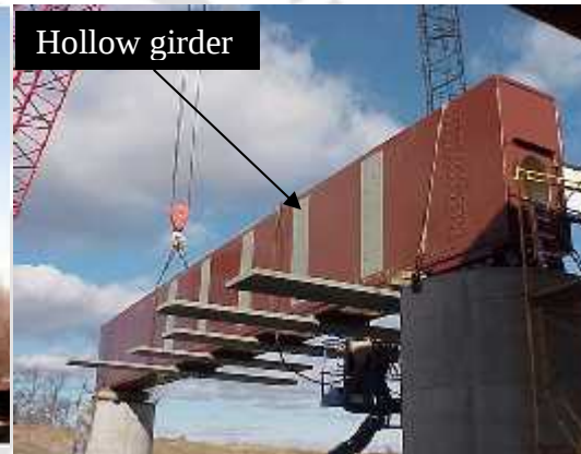
Figure 1.13: Hollow steel beam/steel girder (theconstructor.org)
