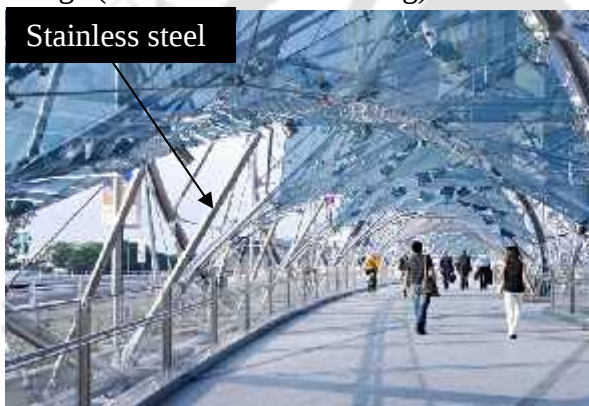
Figure 1.3: Helix Pedestrian bridge ( www.e-architect.co.uk )
