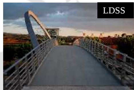
Figure 1. 9: Sant Fruitos Bridge, Spain
