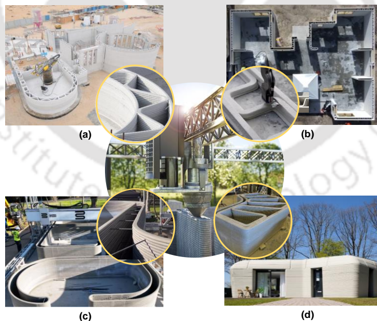
Figure 2.14 Examples of 3D printed housing projects with (structural/ load-bearing) lattice wall Reference: (a) World's largest 3D-printed office building of Dubai Municipality by Apis cor [80], (b) 3D printed model house in Melbourne by Apis cor [81], (c) Austral Australia's first 3D printed amenities block in New south wales by Contour 3D [82], (d) first habitable 3D printed concrete house in Netherland [83].
