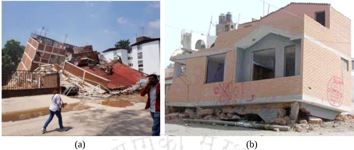
Figure 2.3: Poor performance of CM in: (a) 2017 Mexico City earthquake (Galvis et al. 2020), and (b) 2007 Pisco, Peru earthquake (EERI 2007).
