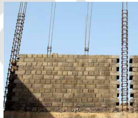
Figure 1.2: Typical confined masonry building: (a) key components of a typical confined masonry building, (b) a single-story confined masonry building with tie-columns, tie-beams, lintel bands, and sill bands (Schacher and Hart (2015), and (c) construction sequence of a masonry wall along with the tie-columns (Jain et al. 2015).
