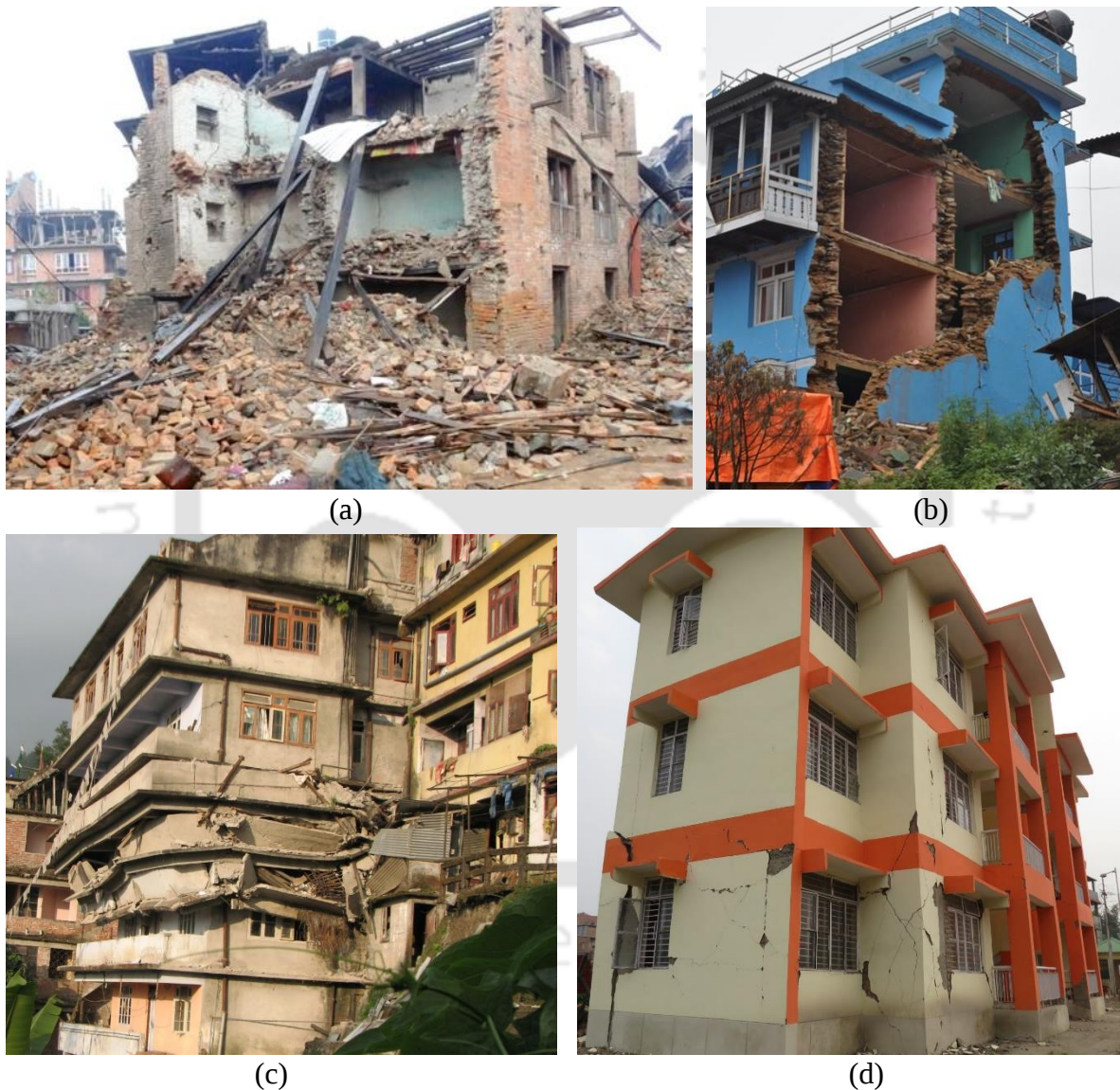
Figure 1.1: Performance of URM and RC buildings in past earthquakes: (a) collapse of a 3-story URM building at Bhaktapur, Nepal (2015 earthquake), (b) out-of-plane collapse of several walls of a 4-story URM building in Dolakha, Nepal (2015 earthquake), (c) pan-cake type failure of intermediate stories of an RC building in Gangtok, Sikkim (2011 earthquake), and (d) poor performance of recently constructed RC building in Imphal, Manipur (2016 earthquake).
