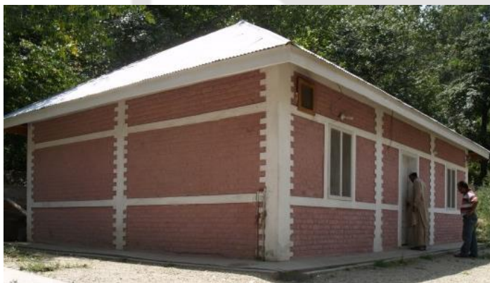
Figure 1.2: Typical confined masonry building: (a) key components of a typical confined masonry building, (b) a single-story confined masonry building with tie-columns, tie-beams, lintel bands, and sill bands (Schacher and Hart (2015), and (c) construction sequence of a masonry wall along with the tie-columns (Jain et al. 2015).
